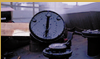
Parabolic antenna still working after use in heavily contaminating double blown bitumen with temperatures over 220 °C (430 °F).
